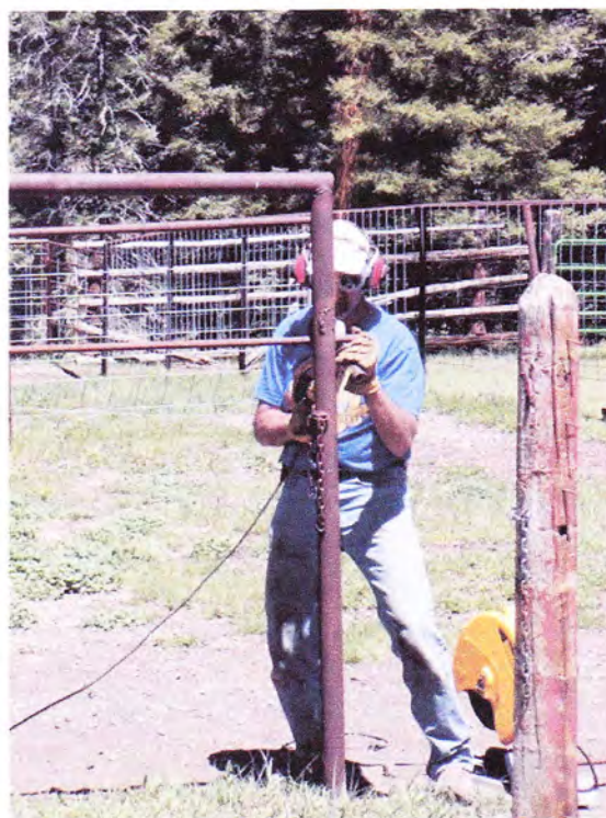
Brad Smith grinding away rust on posts, so Richard K. (below) could weld sucker-rod into place on corrals on west side of barn.
