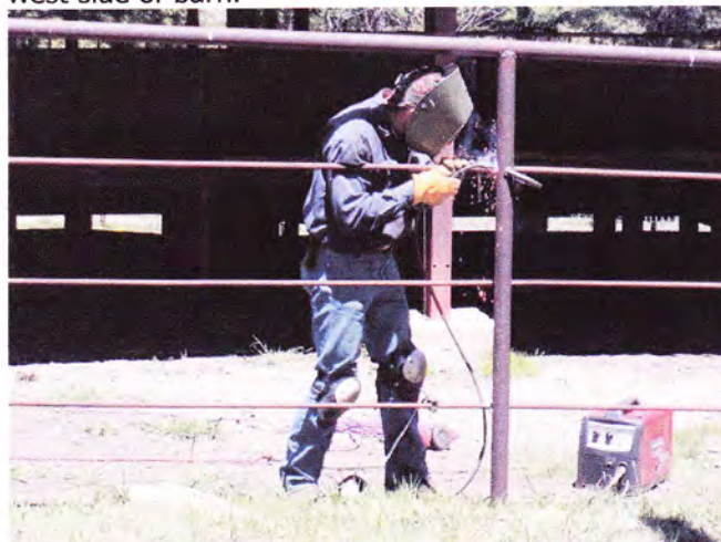
Brad Smith grinding away rust on posts, so Richard K. (below) could weld sucker-rod into place on corrals on west side of barn.
